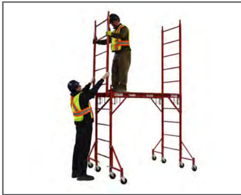
5. When assembling a tower, access the first platform through the hatch. From the ground, have a second person hand components up for the stacked section.
