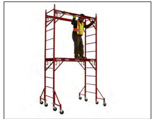
6. Install the two Frames first, then install the two (2) cross members at the desired platform height. Ensure all U-locks are fully engaged and pins are in place prior to installing work platform.
