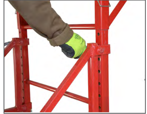
3. Position the outrigger flush onto the end frame, with the castor on the ground. Secure the outrigger in place by tightening the positive engagement locks.
